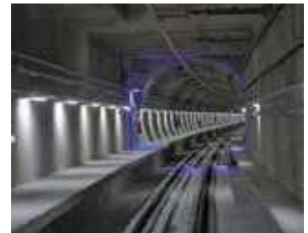
Bosphorus Straits Crossing Railway Tunnel
