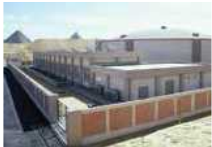
North Pyramid Water Pump Station
