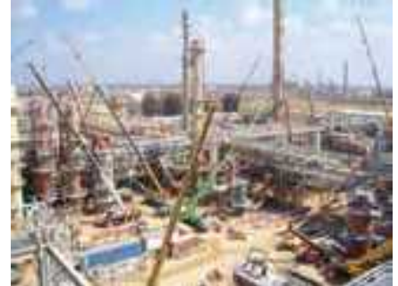
Ethylene Plant Construction
