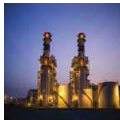
Combined Cycle Power Plant
