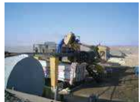
Bituminous sand treatment plant for GPC-JCCP project
