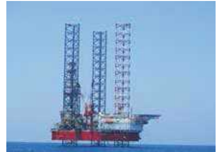
Jack Up Type Drilling Rig "El Qaher II" under operation in the Mediterranean Sea
