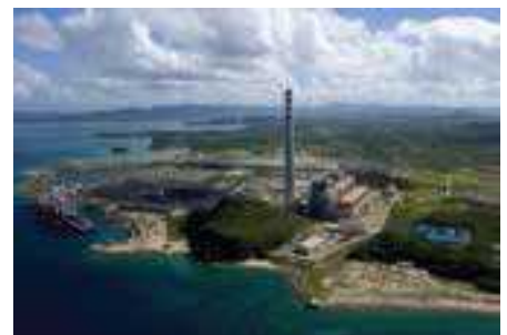
Coal-Fired Thermal Power Plant (IPP)
