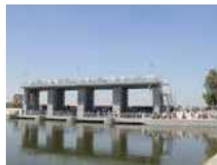
Sakola Regulator on Bahr Yusef Canal SCI carried out design and supervision work
